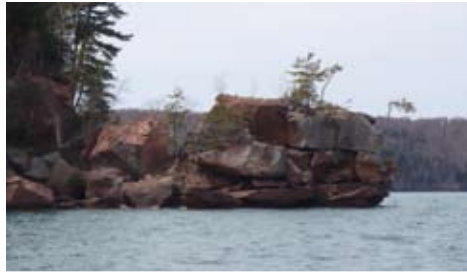
top: Oak Island's "Hole-in-the-Wall" arch in 2004. bottom: Collapsed remains of the arch in April, 2010.
