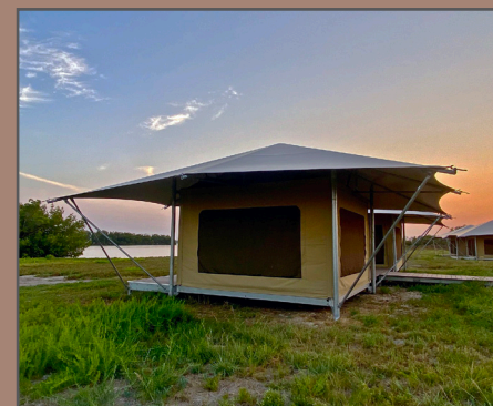
Many national parks are bracing for extreme events. Everglades National Park replaced damaged, brick-and-mortar lodging with a series of canvas “eco-tents” that can be stored during extreme weather events and relocated inland as sea level rises along the coast.
