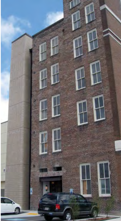
[62] The stair tower at the rear of this commercial building is a compatible new addition.
