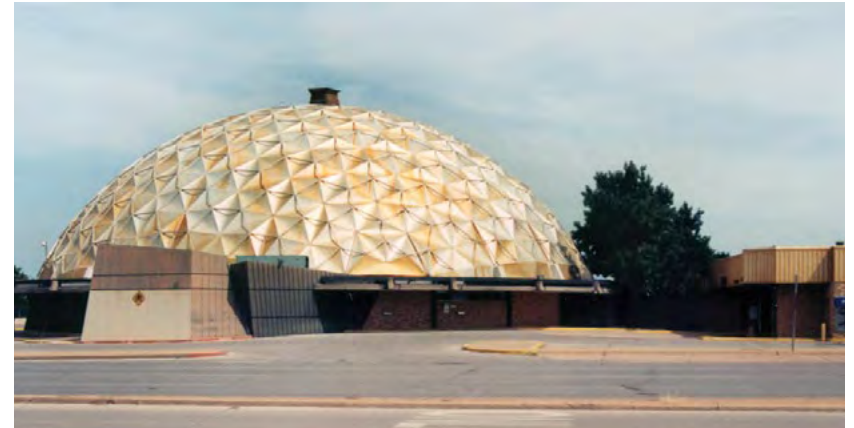
[13] The gold-colored, anodized aluminum geodesic dome of the former Citizen's State Bank in Oklahoma City, OK, built in 1958 and designed by Robert Roloff, makes this a distinctive mid-20th century building.
