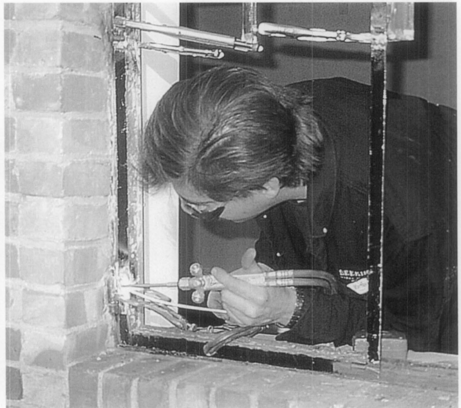
Figure 7. New steel sections were brazed into the historic sash and frame where the windows had previously been altered to fit air conditioning units. Because the replacement pieces came from a stock of salvaged window materials, they matched perfectly the profiles and dimensions of the missing sections.
