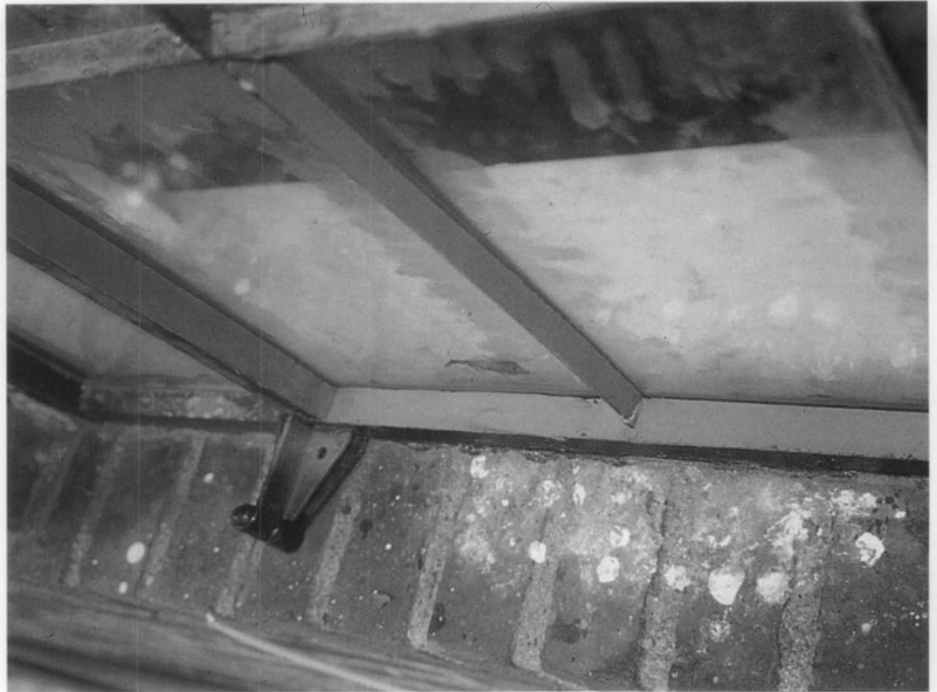
Figure 9. An oil-based putty was used to reglaze the historic casement windows. Painting was undertaken two weeks after reglazing.
