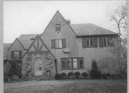
Inappropriate replacement windows dramatically affect the appearance of a historic home that once featured steel casement windows.
