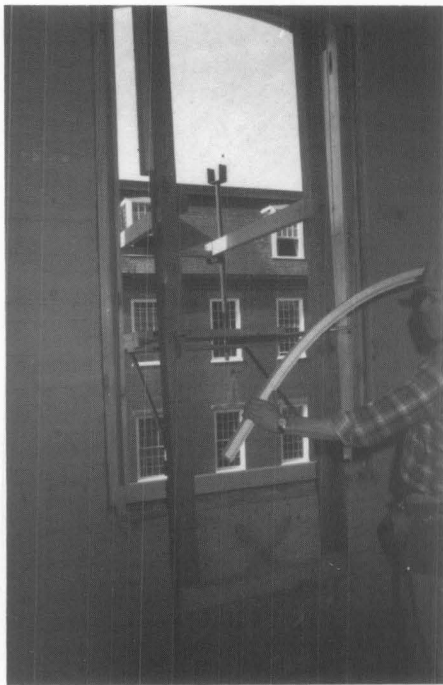
Figure 7. "Gun carriage" (scaffolding) in use by the window re-installation crew who are preparing to replace missing brickmold with replacement made by the millwork shop. Note saw kerfs used to create arc in molding for use in the window head (same method as used in the original molding). Photo: Christopher Closs
