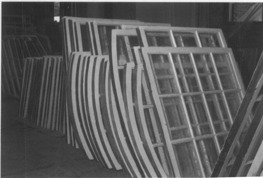
Figure 5. Repaired sash primed and awaiting reinstallation. Glass was cleaned of smudges after final installation. Photo: Christopher Closs
