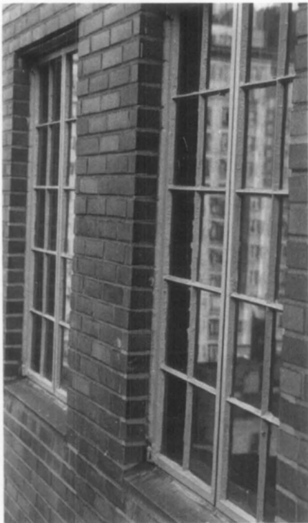
Figure 7. The dark frame color and careful installation of the interior storm window resulted in little visual impact on the exterior appearance of the building. Photo: Charles Fisher.
