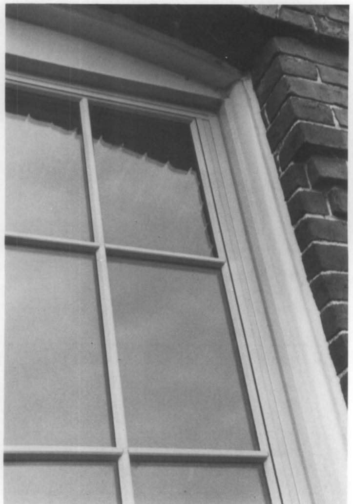
Figure 4. A custom-extruded aluminum pan was installed, duplicating the brick molding detail and, at the head of the frame, custom bent to follow the segmental curve of the masonry opening. Photos: Charles Fisher
