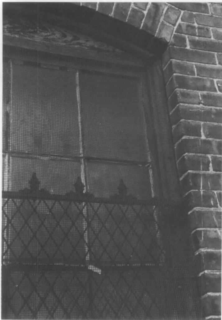
Figure 4. A custom-extruded aluminum pan was installed, duplicating the brick molding detail and, at the head of the frame, custom bent to follow the segmental curve of the masonry opening. Photos: Charles Fisher
