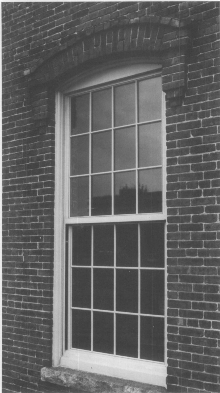
Figure 7. Replacement window after installation. Photo: Charles Parrott
