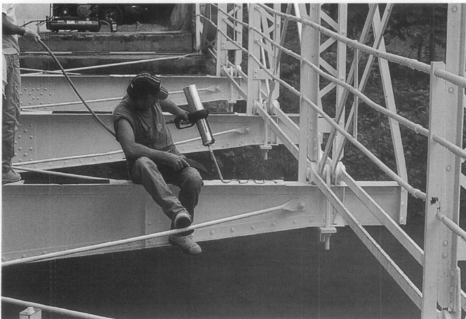
Figure 9. A worker applied adhesive to the floor beams where each of the bearing pads would be positioned. Four pads were installed on each floor beam to cushion the deck, evenly distribute loads to the floor beam and provide a secure fit between beam and deck.
