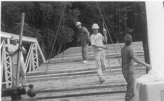
Figure 11. As the deck was lifted off the trailer and onto the floor beams, workers wedged timbers and bars along the sides to prevent the deck from damaging the truss and to help place the deck in position.
