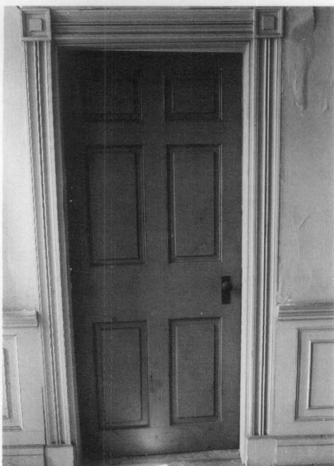
Figure 16. This residential door shows how scuffed and abraded interior painted surfaces can become over time, particularly if the feature is in a high-use area. In the preservation project, the door was simply cleaned and repainted the same color. Photo: Robert M. Smith, Jr.
