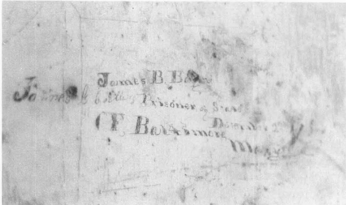
Figure 12. When discovered, important examples of history such as this pencilled Civil War graffiti should be preserved. A conservator can easily clean the area, then apply a protective coating. The history this hand-written message possesses is well worth the sacrifice of surface uniformity, even if it interrupts a freshly painted surface. Photo: Kaye Simonson.
