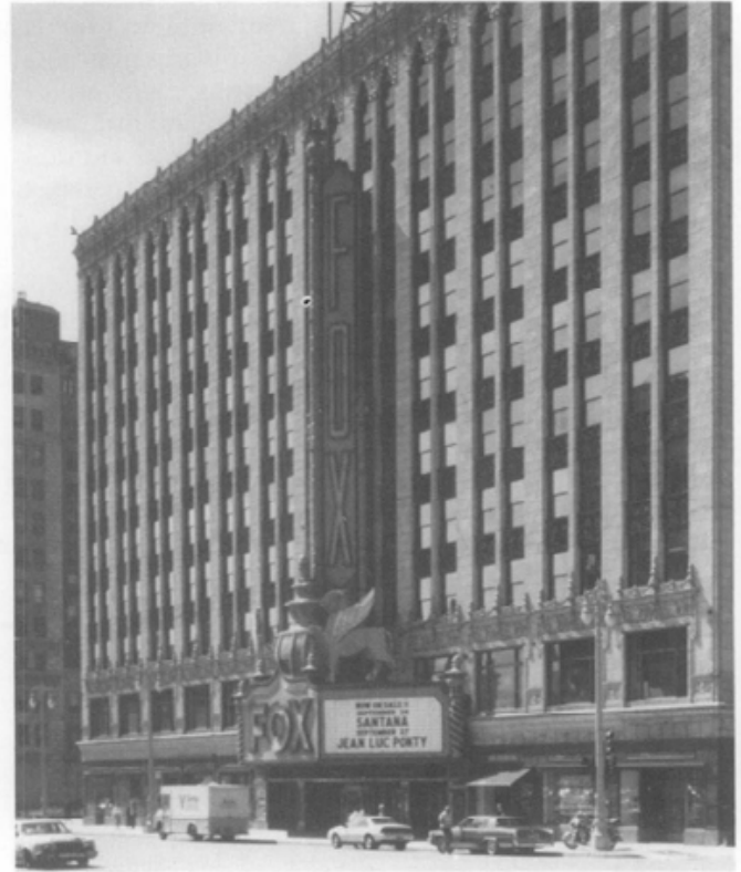
3. The circa 1928 Fox Theater in Detroit, designed by C. Howard Crane, was one of the earliest twentieth century buildings to provide air conditioning to its patrons. The early water-cooled system was recently restored. Commercial and highrise buildings of the twentieth century were able, mostly through electrical power, to provide sophisticated systems that integrated many building services. Photo: William Kessler and Associates, Architects.
