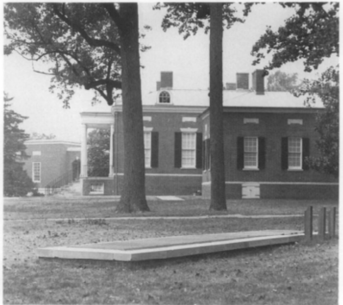
11. During the restoration of this 1806 National Historic Landmark (photo a), a new climate control system was installed. The architects removed all the earlier mechanical equipment from the house and installed new equipment in a 30' x 40' concrete vault located underground 150 feet from the house itself (photo b). Only conditioned air is blown into the house reusing much of the circa 1930s ductwork. Photos: Thomas C. Jester.
