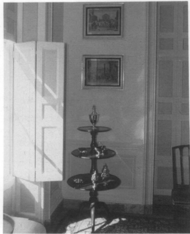
f. Homewood, Baltimore, MD. This elegant circa 1806 residence is now a house museum. The registers for the forced air ducted system seen behind the table legs, are grained to blend with the historic baseboards. The HVAC system uses a water/air system where chilled water and steam heat are converted to conditioned air. Photo: Courtesy Homewood Museum, Johns Hopkins University.
