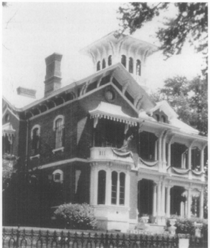
2. Nineteenth century buildings continued to use architectural features such as porches, cupolas, and awnings to make the buildings more comfortable in summer, but heating was greatly improved by hot water or steam radiators. Photo: NPS Files
