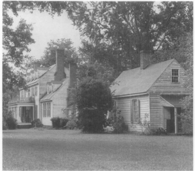
1. Eighteenth century and later vernacular architecture depended on the siting of the building, deciduous trees, cross ventilation, and the placement of windows and chimneys to maximize winter heating and natural summer cooling. Regional details, as seen in this Virginia house, include external chimneys and a separate summer kitchen to reduce fire risk and isolate heat in the summer. Photo: NPS Files.
