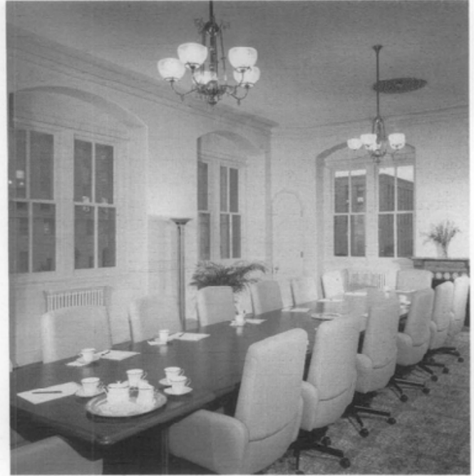
c. Conference room, Auditors Building, Washington, D.C. The historic steam radiators were retained for heating. The cast iron ceiling register was retained as a decorative element, but made inoperable to meet fire codes. Photo: Kenneth Wyner Photography courtesy of Notter Finegold + Alexander Inc.
