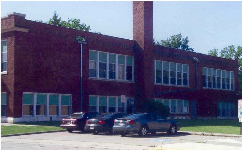
Top: Rear façade of school prior to rehabilitation.
