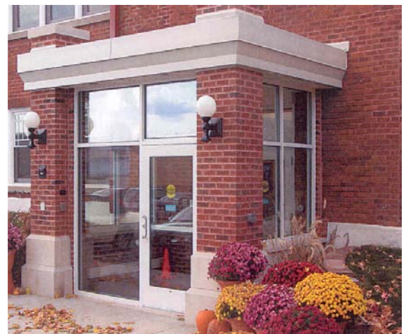
Bottom: New accessible entrance. The same brick and limestone were used for the addition, while contemporary-styled windows and doors help to differentiate the new construction.
