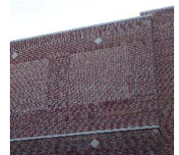
Below: Detail of fly loft showing compatible brickwork.
