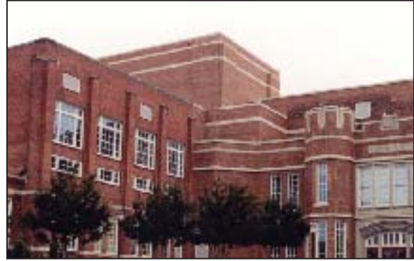
Rear elevation of the school showing new fly loft redesigned to meet the Standards.
