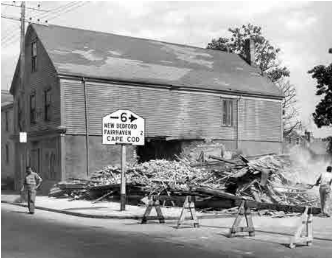
Fig. 6.17. St. Ambrose African Orthodox Church, Kempton Street, 22 July 1960. A section of the church's west wall caved in when a building next door, condemned and then being removed, collapsed, twisted, and struck the church. Courtesy Spinner Publications.
