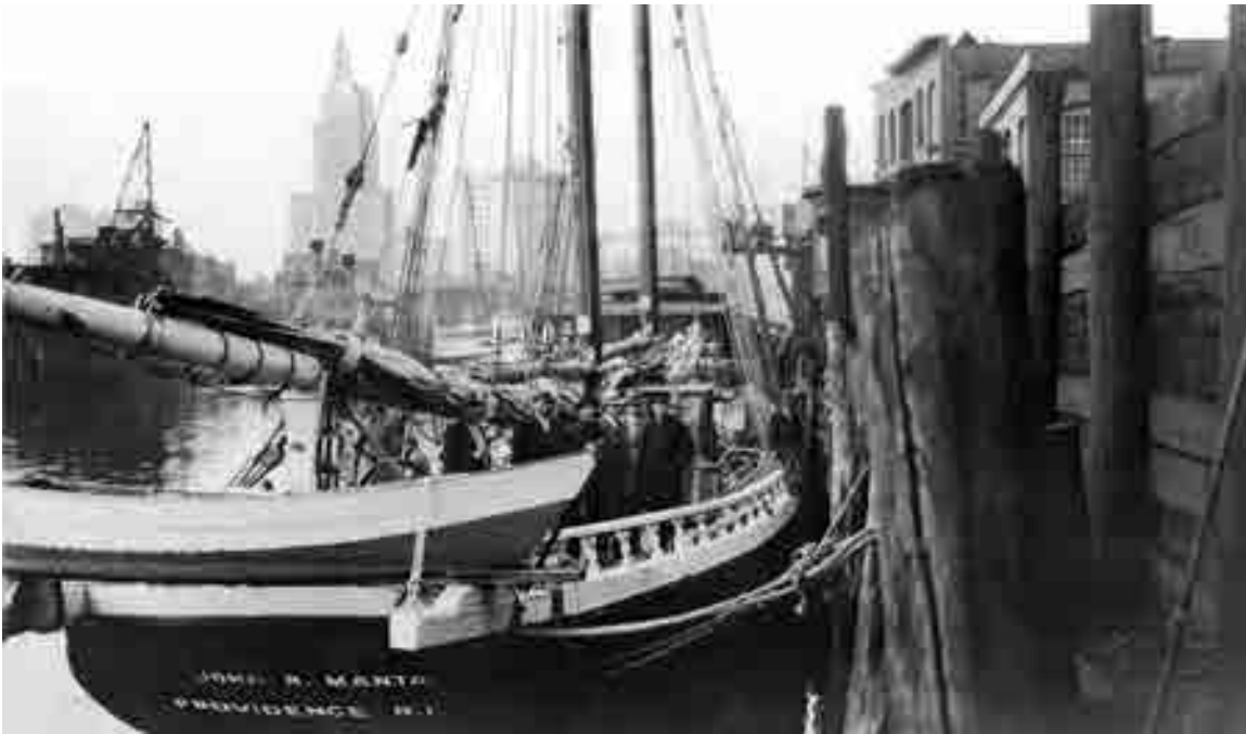
Fig. 11.8. The former whaling schooner John R. Manta as a Cape Verde packet, at dock in Providence, 1927–34. New Bedford’s last successful whaling voyage was the 1925 cruise of the John R. Manta under master and owner Antonio J. Mandly. In June 1927 Mandly sent master Joseph F. Edwards out in the vessel, but it returned to port heavily damaged by gales three weeks later. By the fall Mandly sold the Manta to Providence buyers, who entered it into the packet trade. The vessel was lost with all crew and passengers in the Atlantic in the winter of 1934-35. Courtesy New Bedford Whaling Museum.
