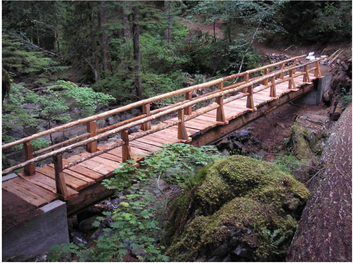
New bridge over Laughingwater Creek on the Silver Falls Loop Trail.
