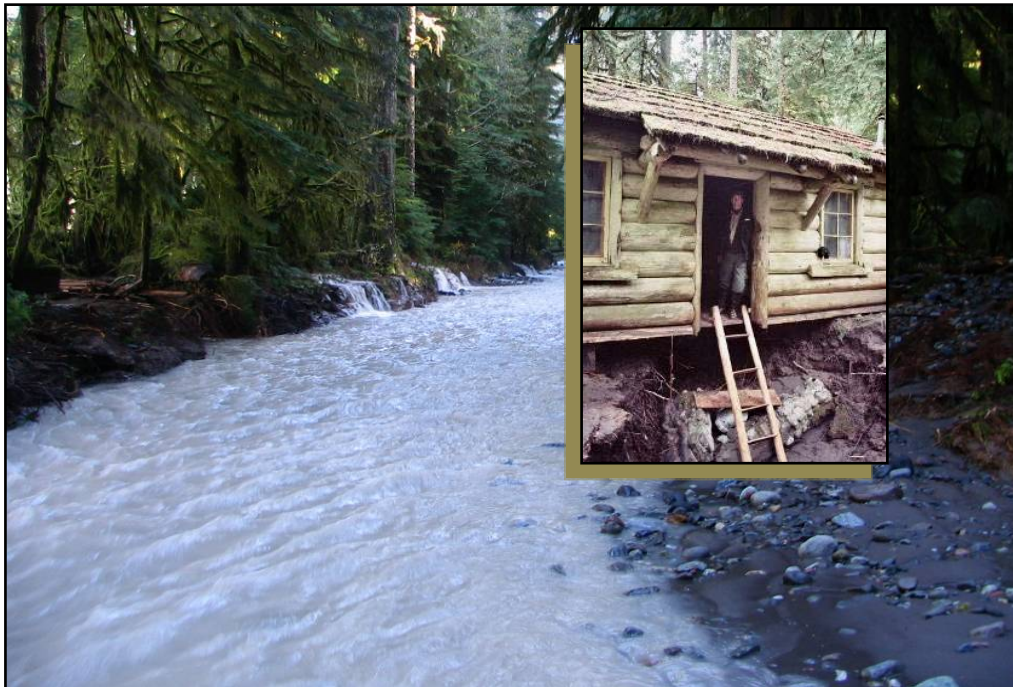
More than two miles of road were destroyed along the Carbon River. Ipsut Creek cut a deep channel directly beneath the historic Ipsut Creek Patrol Cabin.
