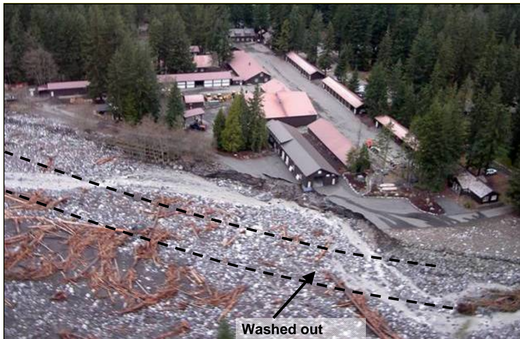
Re-establishment and improvement of flood protection structures at Longmire are underway with the Longmire levee now complete.
