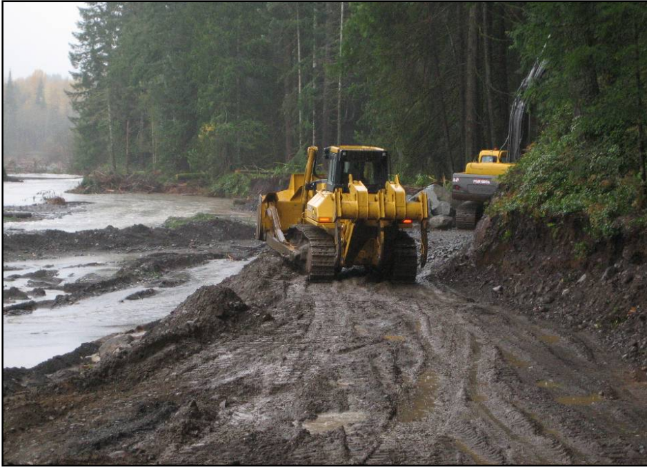
At Sunshine Point, construction began on a replacement road on November 8, 2006.
