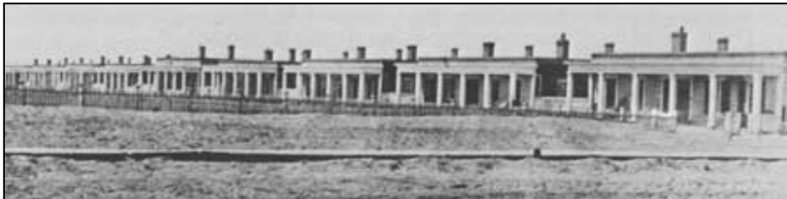
Officers' row, Fort Union, in the 1870s. The nine quarters were numbered from right to left. The commanding officer's quarters were No. 5 in the center. U.S. Signal Corps Photo No. 88020, courtesy National Archives.
