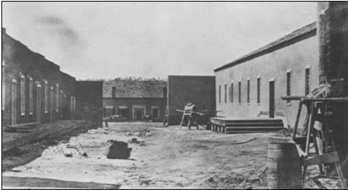
View between two Fort Union Depot storehouses, probably in 1866, with the depot quartermaster office in background. The storehouse on the right was nearing completion; note scaffold, bucket, and trowel. It was the only large storehouse with a gable-style, shingled roof. U.S. Signal Corps Photo No. 87992, courtesy National Archives.
