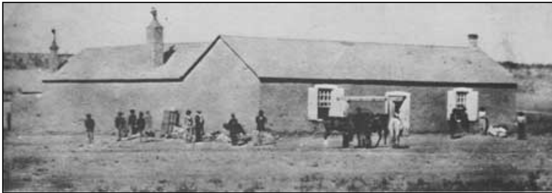
Post trader's store at Fort Union, probably late 1860s. U.S. Signal Corps Photo No. 87966, courtesy National Archives.
