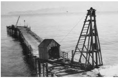
The pier with pile driver in operation.
