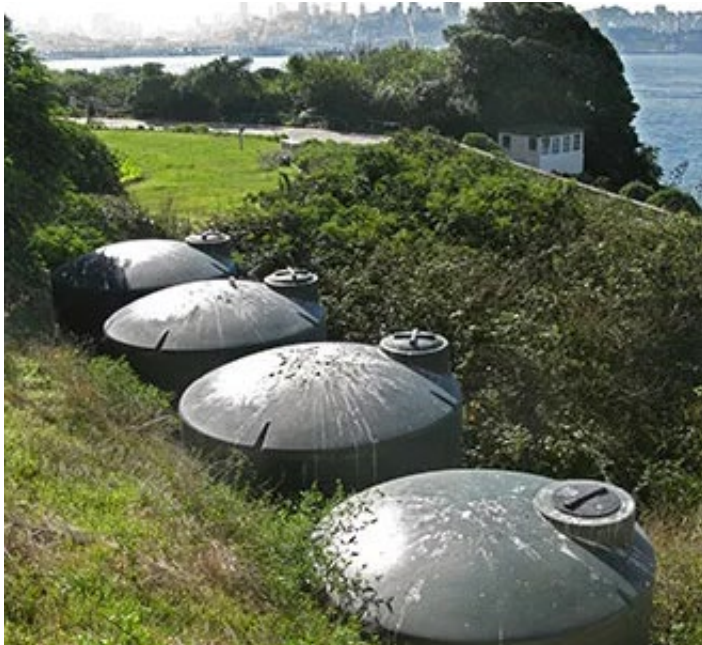
Alcatraz Island uses a rainwater catchment system to capture water for landscaping the historic gardens on the island. Credit: NPS
