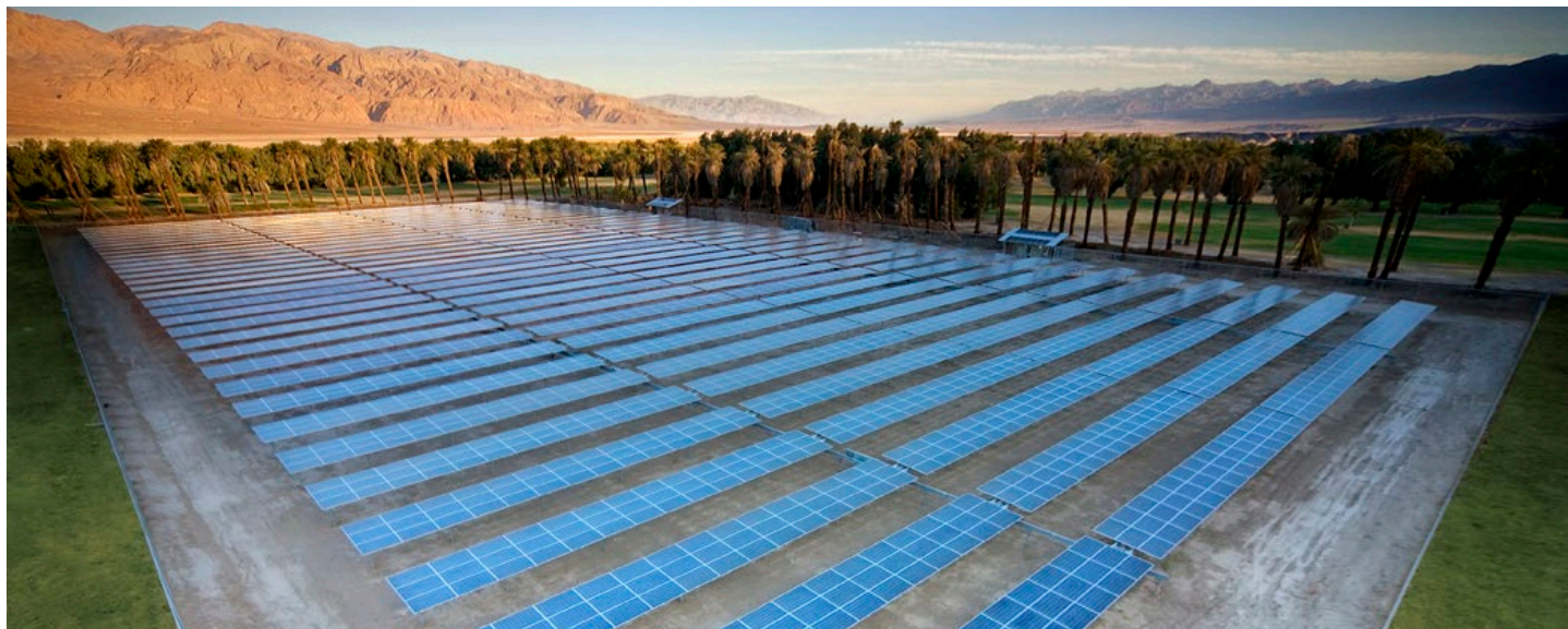
Solar panels at Furnace Creek in Death Valley National Park. Credit: NPS
