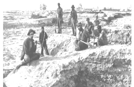
Soldiers constructing earthworks during the war
