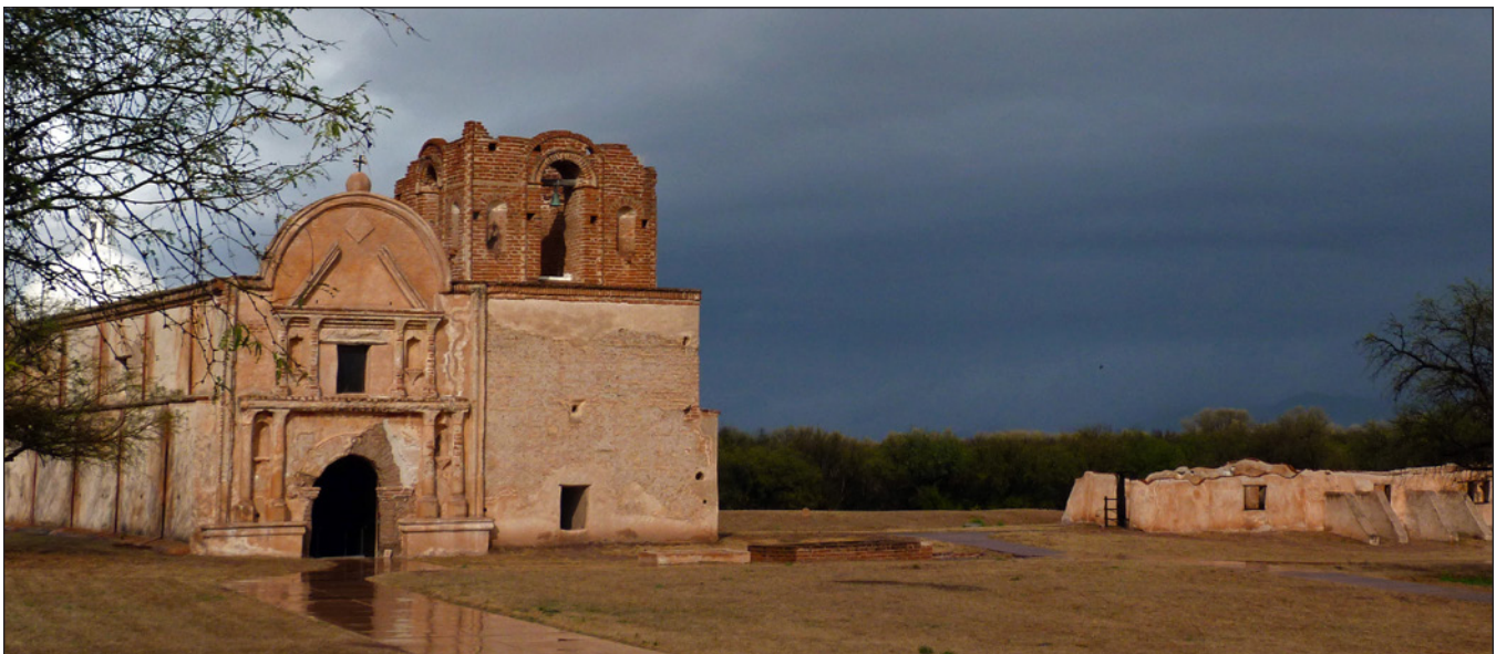
The mission church at Tumacácori National Historical Park is one of many adobe structures across the National Park System. Adobe is susceptible to damage from warming temperatures and changing precipitation patterns driven by climate change.
