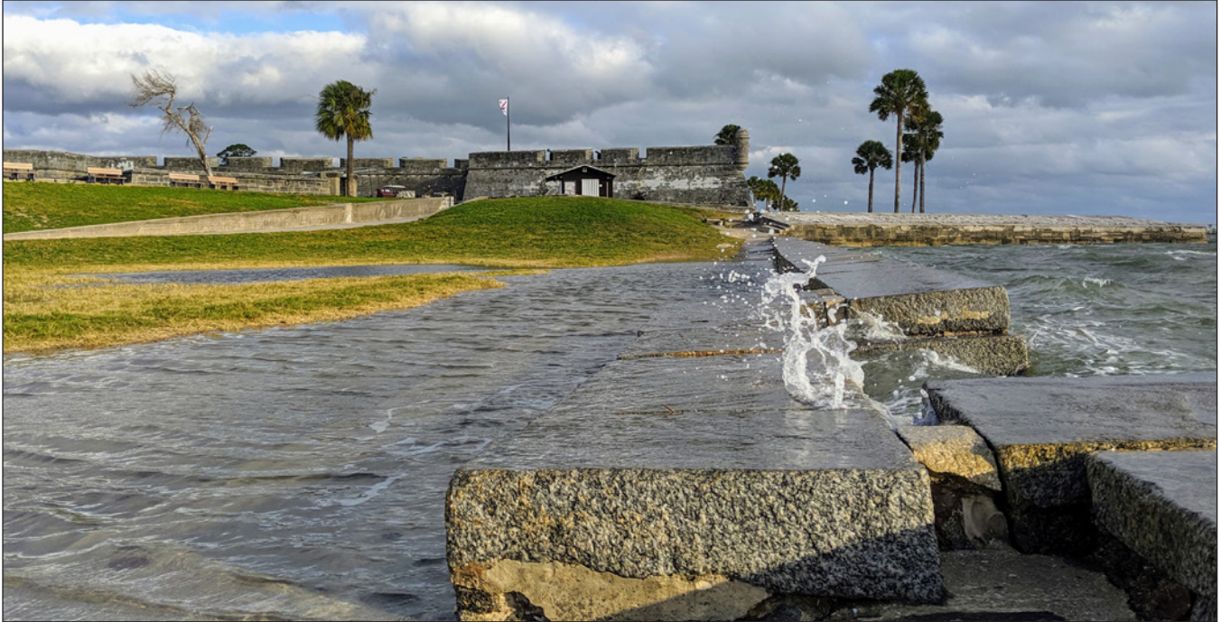
A 2022 assessment found roughly one-third of all building and transportation assets at Castillo de San Marcos National Monument are highly vulnerable to coastal hazards and sea level rise.
