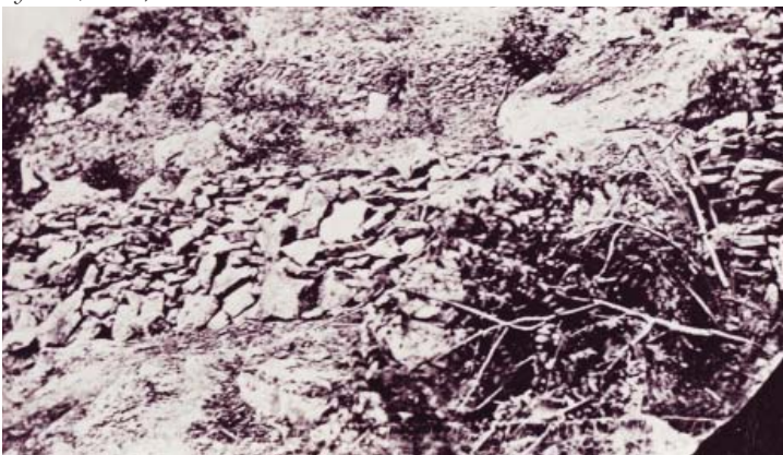
Figure 5.06. Stone breastworks as they appeared immediately following battle. Breastworks were hastily erected during battle to provide immediate protection for defending Union troops. Photograph by O'Sullivan (GNMP General Historic Photographic Prints GETT 41135 #SF-2B-2095).
