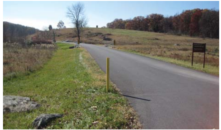
Figure 3.03. Crawford Avenue, looking south (Photo by RHI, 2010).
