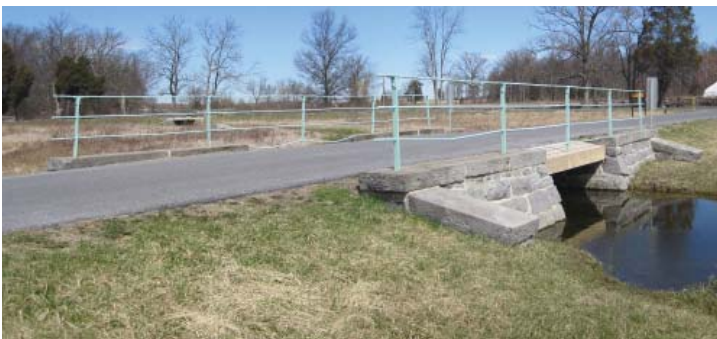
Figure 3.11. War Department Era bridge over Plum Run at Crawford Avenue, near the intersection with Wheatfield Road (Photo by RHI, 2011).
