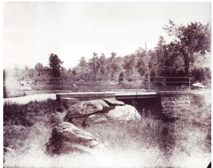
Figure 2.35. View of completed bridge on Warren Avenue over Plum Run. Photograph by Tipton, 1903. (GNMP Tipton Photographic Prints GETT 41136 #3020).
