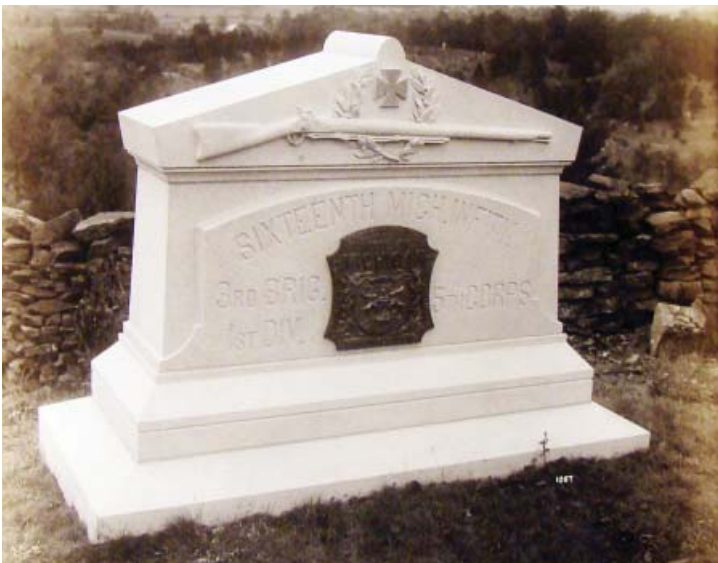
Figure 5.07. Rehabilitated stone breastworks behind the 16th Michigan Infantry Monument. Although more structurally sound than the original construction, the rehabilitated breastworks often do not convey the haste with which the original breastworks were constructed. Photograph by Tipton, 1889 (GNMP Tipton Photographic Prints GETT 41136 #5036).
