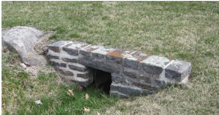
Figure 3.88. War Department Era square-topped stone culvert (Photo by RHI, 2011).
