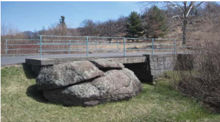
Figure 3.12. War Department Era bridge over Plum Run at Warren Avenue, near the intersection with Crawford Avenue (Photo by RHI, 2011).
