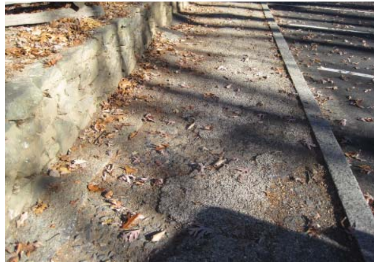
Figure 3.16. Granite curb and asphalt sidewalk at the Sykes avenue parking area (Photo by RHI, 2010).
