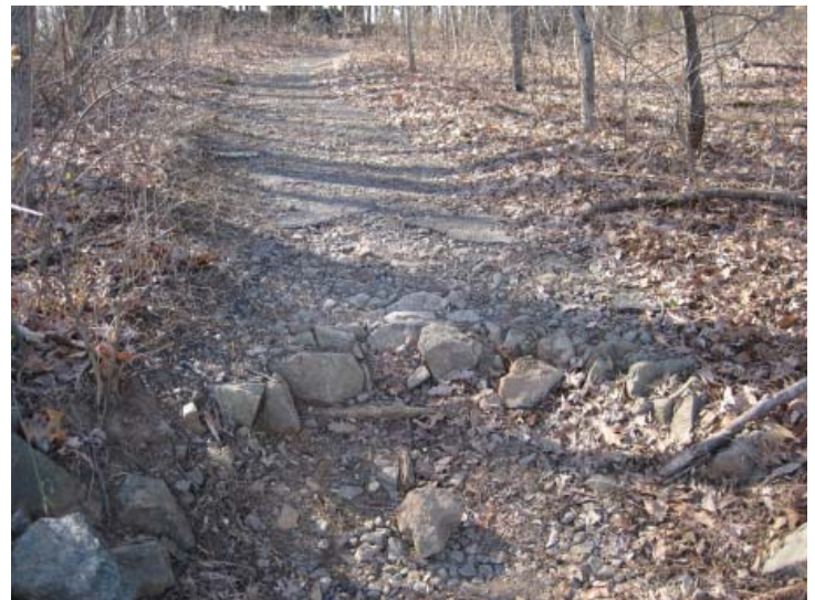
Figure 3.23. The maintained horse trail that traverses Little Round Top's eastern slope utilizes a portion of the historic Sykes Avenue alignment. At the intersection with Wheatfield Road, a portion of the Telford road base and asphalt paving is still apparent. (Photo by RHI, 2011).
