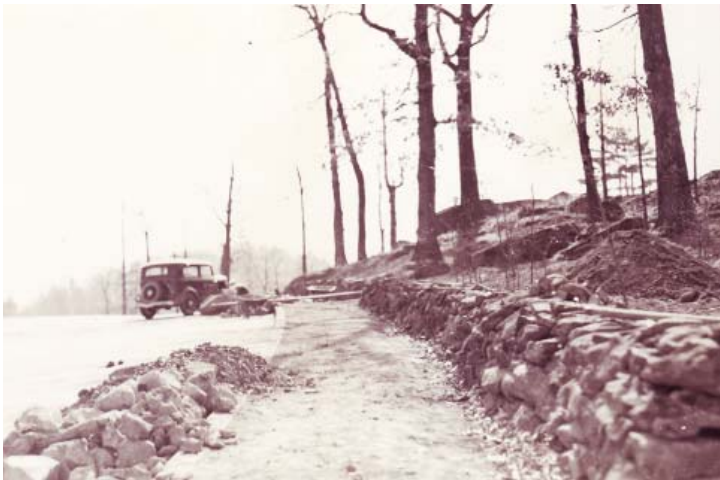
Figure 2.42. Construction of walkways and retaining wall at the Sykes Avenue parking lot on Little Round Top, ca. 1936-1937 (GNMP General Historic Photographic Prints GETT 41135 #SF-30W-093).
