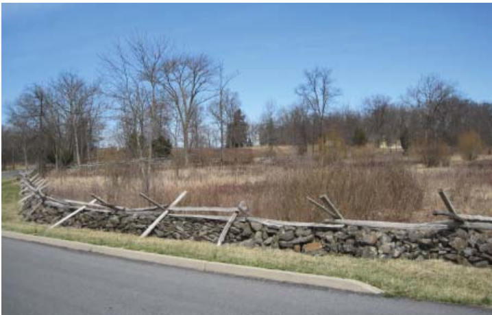
Figure 5.05. Fences, such as this stone fence with rider along Wheatfield Road, are regularly restored in their original locations, using historic methods and materials. Restoration projects like this are crucial to providing visitors with the most accurate interpretive experience possible. (Photo by RHI, 2010).
