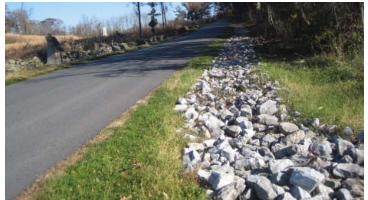
Figure 3.92. Rip-rap lined drainage channel along Wheatfield Road (Photo by RHI, 2010).
