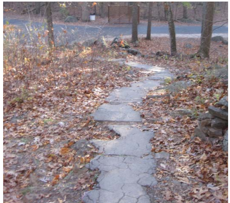
Figure 3.18. Asphalt path leading from the top of Vincent Spur to Wright Avenue (Photo by RHI, 2011).
