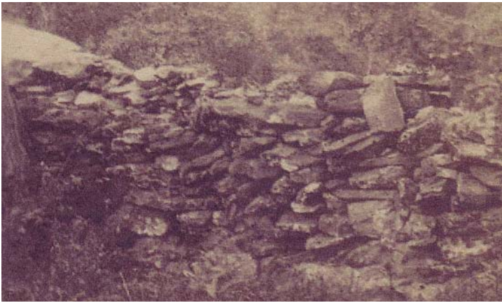
Figure 6.04. Reconstructed breastworks on Little Round Top, circa 1880. Breastworks constructed during battle would have been much simpler than the high stone wall depicted here. The need to interpret this key battle-era feature was recognized early, however, and breastworks have been continually rebuilt throughout the park's history (Susan Boardman Collection of Historic Stereographic Views #SV-713).
