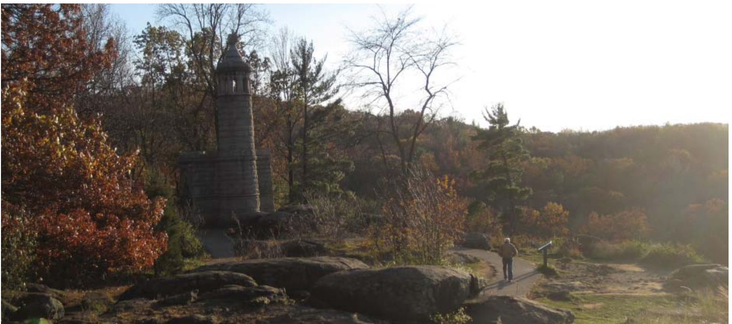
Figure 3.121 Looking south along the summit of Little Round Top toward the 44 th and 12 th New York Infantry Monument, within the Core Interpretive Character Area. Note the degradation to the landscape on either side of the asphalt path (Photo by RHI, 2010).
