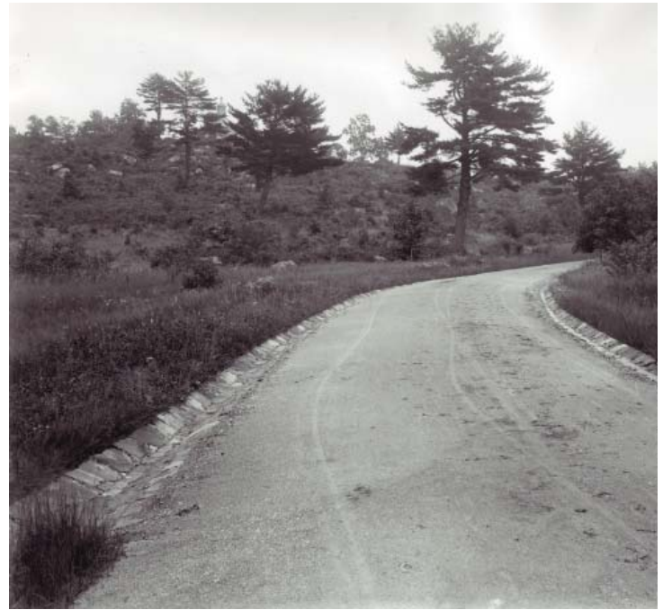
Figure 2.32. Detail of flagstone gutter paving on Warren Avenue. Photograph by Tipton, 1904 (GNMP Tipton Photographic Prints GETT 41136 #3140).
