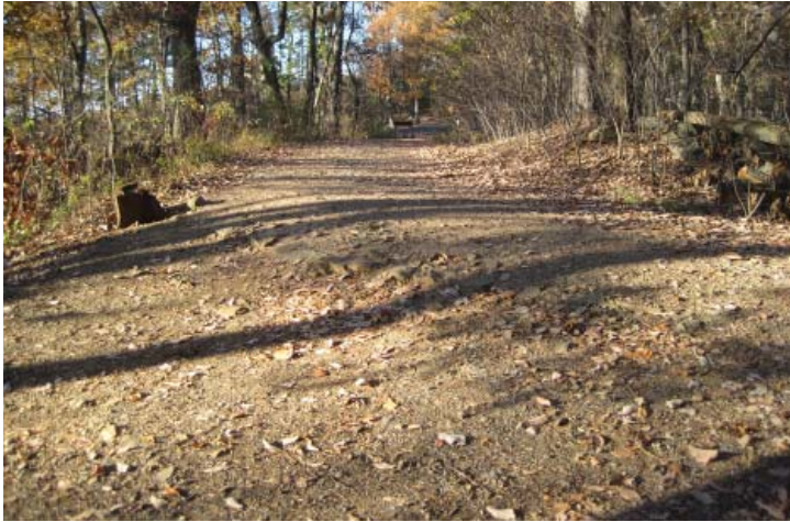
Figure 3.10. Chamberlain Avenue road trace. All that remains is the Telford base (Photo by RHI, 2010).
