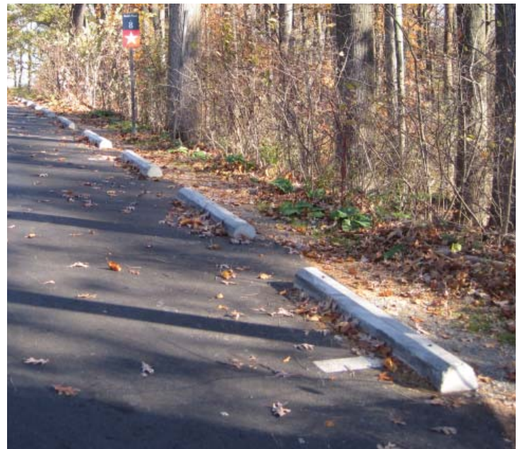
Figure 3.17. Concrete wheel stops prevent vehicles from driving off the side of Sykes Avenue and down the adjacent slope. (Photo by RHI, 2010).
