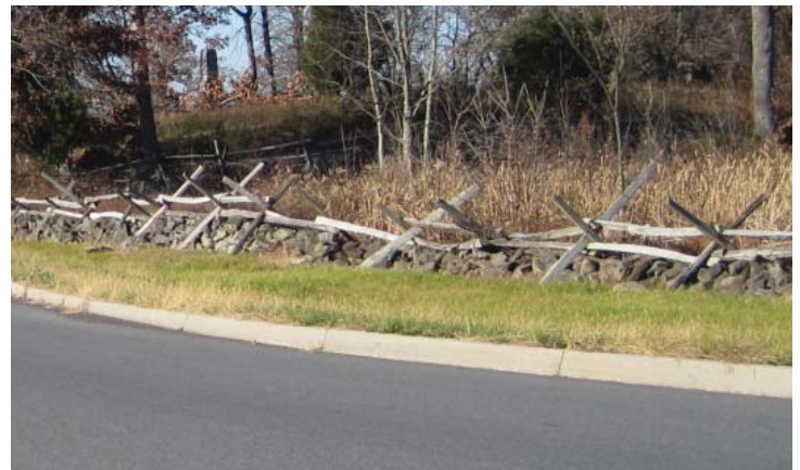
Figure 3.15. Concrete curb along the northern edge of Wheatfield Road. (Photo by RHI, 2010).
