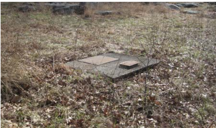
Figure 3.80. Concrete well cap near the asphalt pull-off on Warren Avenue (Photo by RHI, 2011).
