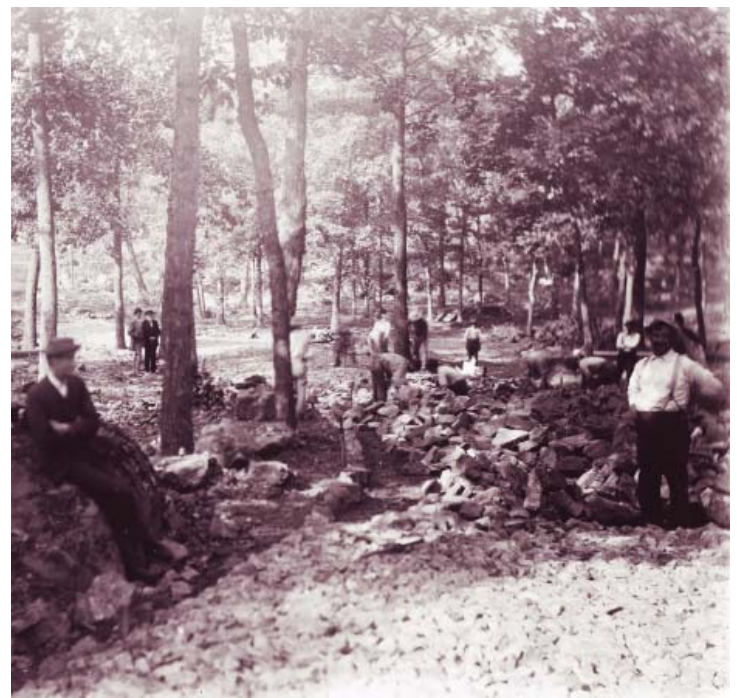
Figure 2.30. Construction of Sykes Avenue at the foot of Big Round Top, showing men laying base stones, looking in the direction of Vincent Spur. Photograph by Tipton, 1897 (GNMP Tipton Photographic Prints GETT 41136 #3098).
